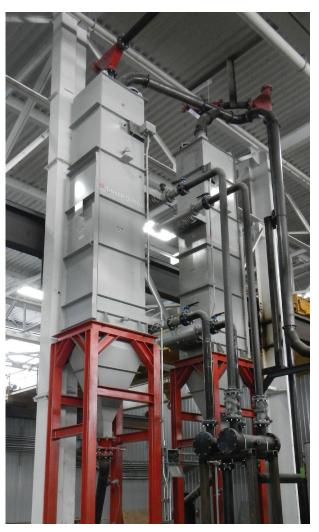
The modular design and vertical orientation of today's plate heatexchangers require minimal floor space, which, in turn allows for seamless retrofits to existing plants with minimal CapEx and infrastructure modifications. (Solex Thermal Science)
